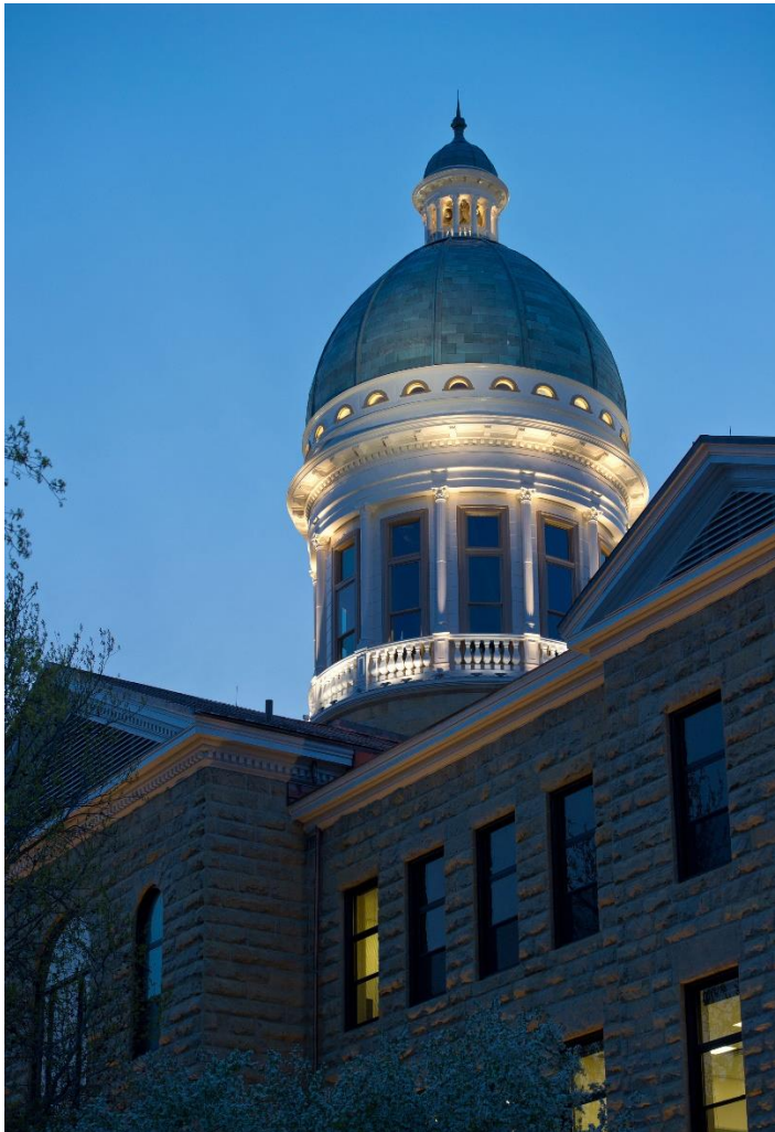
Old Main has been a landmark at Augustana College since 1883. The building is listed on the National Register of Historic Places.
